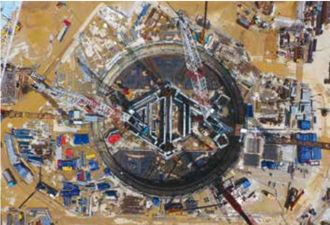
Main tower piling work - 16 August 2016
